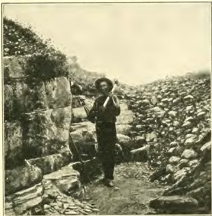
FIG. 128. Indian miner breaking up the exposed margin of the pipestone layer.
